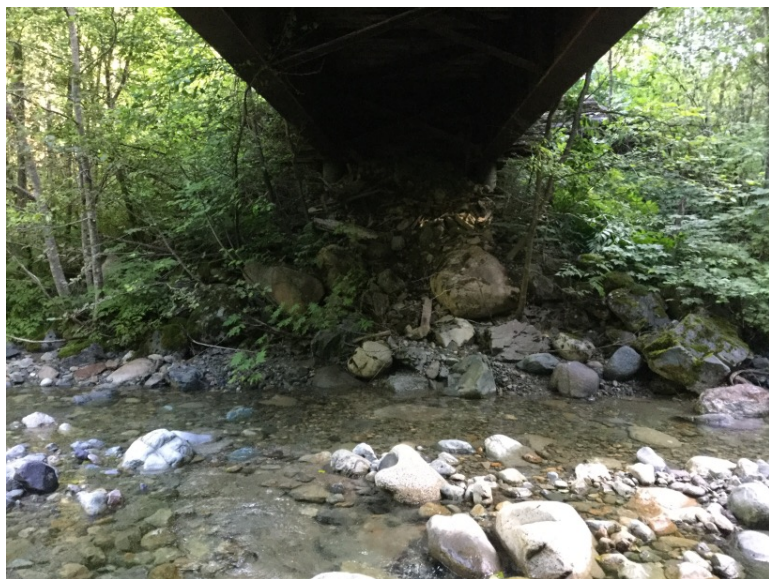
Right Bank Abutment when facing downstream
