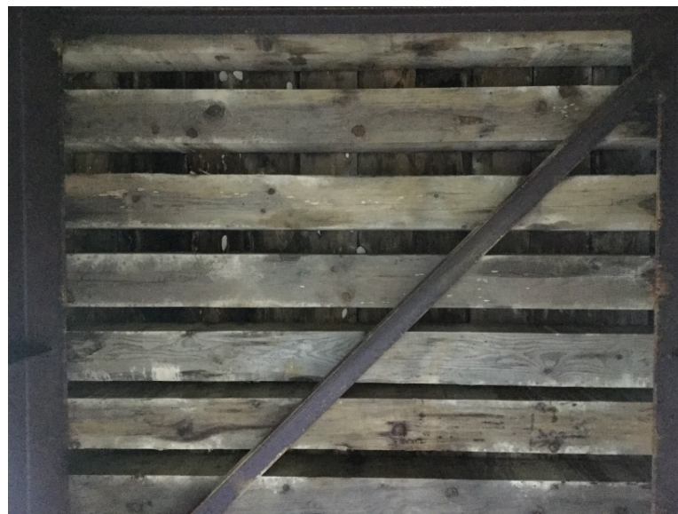
Deck from underneath
