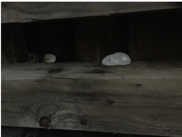
Small fruiting body present on single tie and at various locations of subdeck - typical size shown
