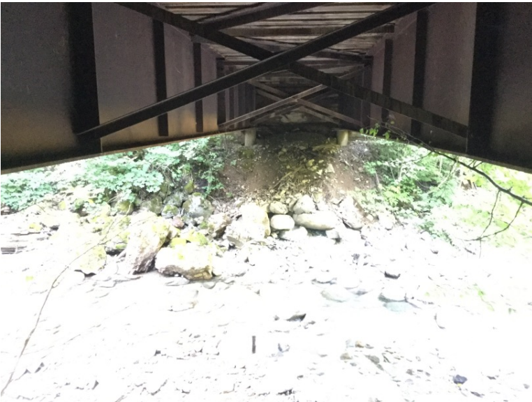
Left Bank Abutment when facing downstream
